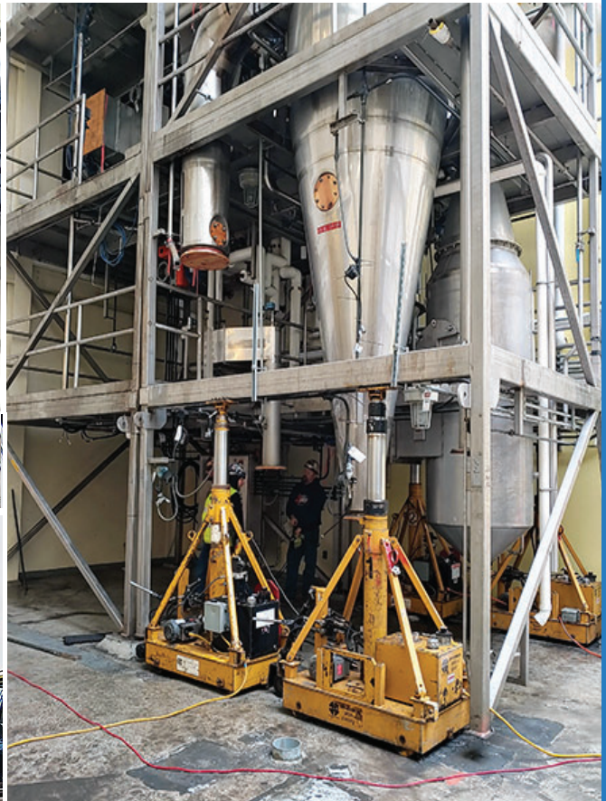
Above: We utilized yellow hydraulic gantry jacks to boost these processing units so that they could be lifted with a 350 ton crane. Left: You can see the units being lifted and put onto a lowboy for transport to their new locations.
